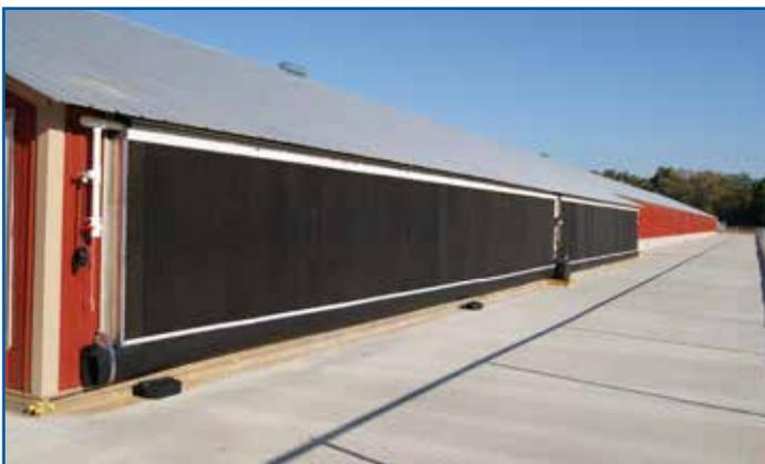
**Figure 117:** Pad cooling with tunnel ventilation.
