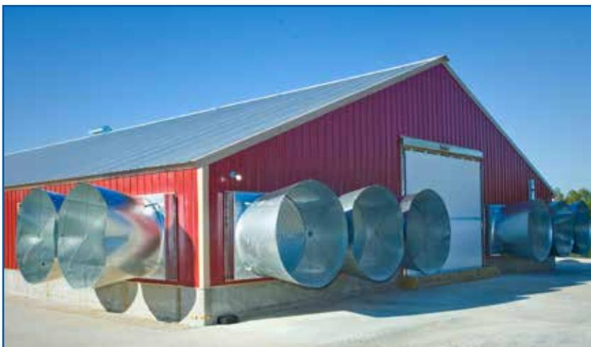
The system uses fans (usually 122 cm [48 in] or 127 cm [50 in]) at one end of the house and air inlets at the other end. High volumes of air are drawn down the length of the house, exchanging the air in the house in a short time (**Figure 113**).
