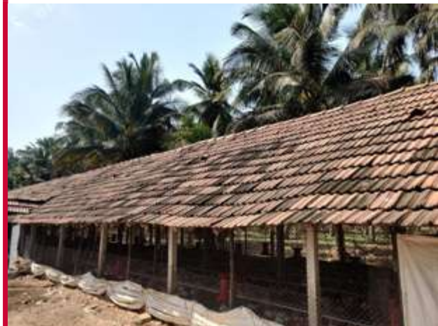
Figure 95 Example of typical open-sided housing.
