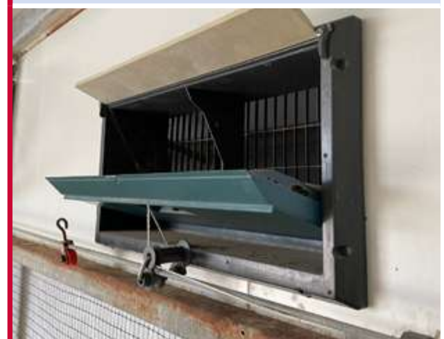
Figure 100 Example of a good-quality air inlet.
