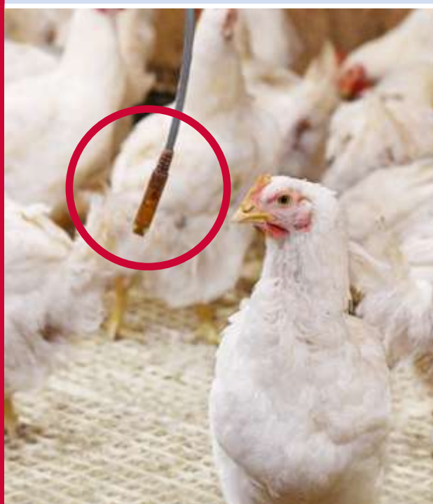
Figure 17 Correct location for temperature/humidity sensors.
