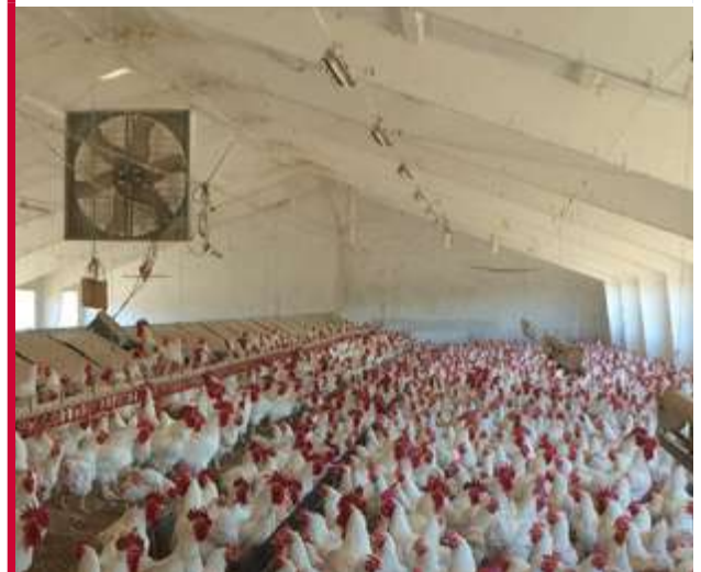
Figure 96 Circulation fans in an open-sided/naturally ventilated house.
