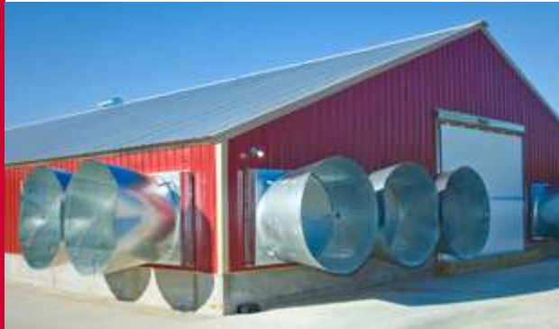
Figure 107 Example of a typical tunnel-ventilated house.
