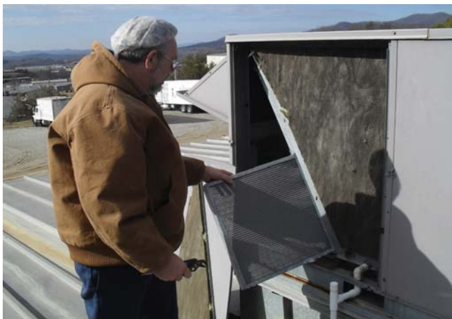
Figure 1: Maintenance and cleaning should be carried out on any equipment that can affect the performance of the hatchery. This includes ancillary equipment such as air handling equipment.
