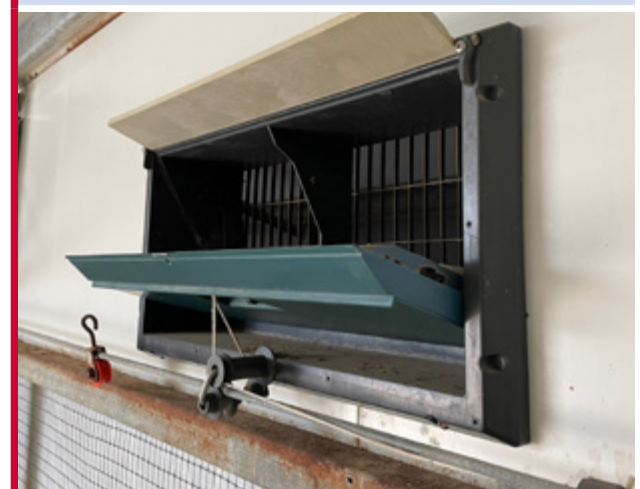
Figure 100 Example of a good-quality air inlet.
