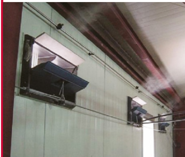
Figure 112 Example fogging system for a cross-ventilated house.
